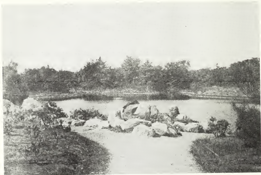
The Rockery under construction
